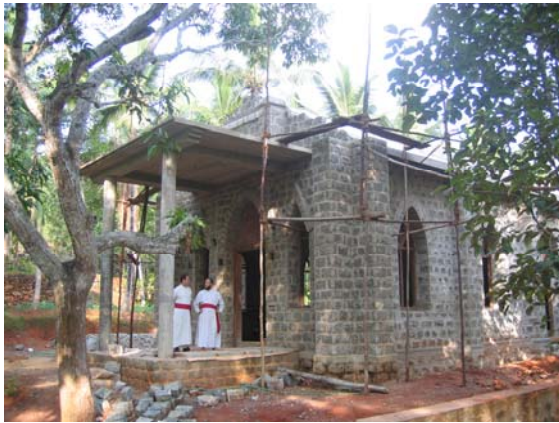
Summer 2005: Frs. Blute and Summers surveying the work already completed.
