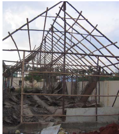
Right: Deo Gratias! The disassembling of the former shed "chapel" at the priory. For more than two years the parish Mass was held in this primitive structure. All the faithful and especially the priests were happy to see it demolished.
