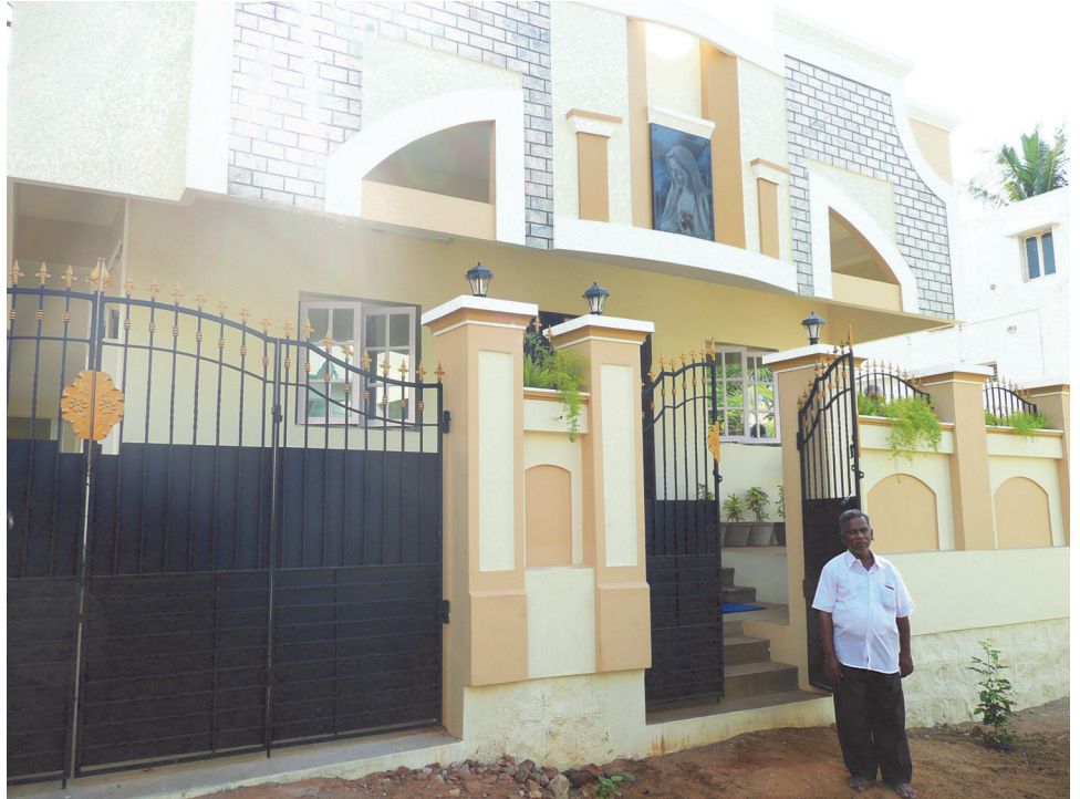
Mr. John Sarto, housekeeper and factotum, stands in front of the interesting façade of the recently completed St. Joseph's Chapel, Trichy.
