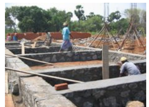
...but were finished in no time.
