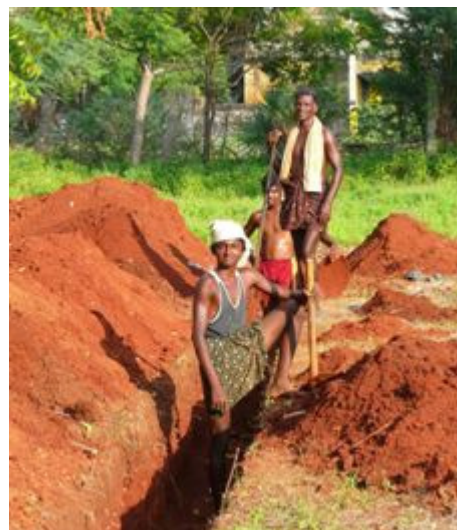
Foundations were dug the hard way...
