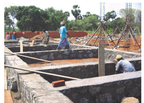
...but were finished in no time.
