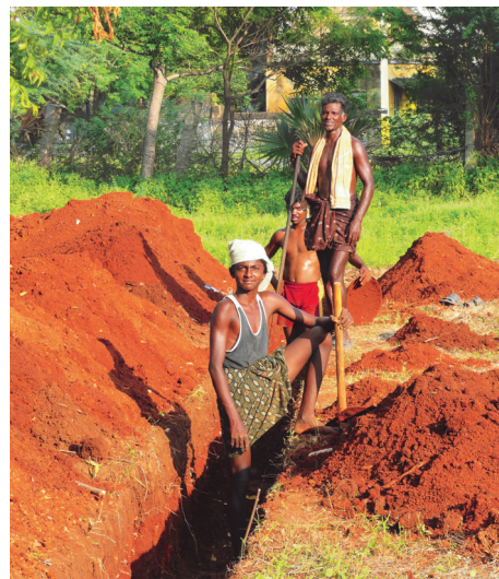
Foundations were dug the hard way...
