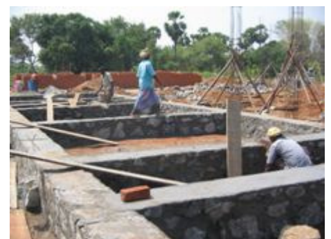
...but were finished in no time.
