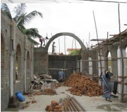
Another building site. Chennai.
