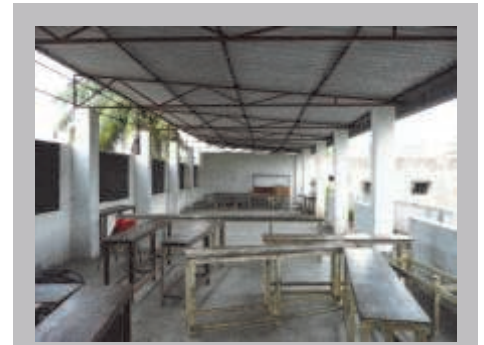
St. Anthony's Chapel (see opposite page, far left) was built on the roof of St. Anthony's School. This is what it looked like before construction started.
