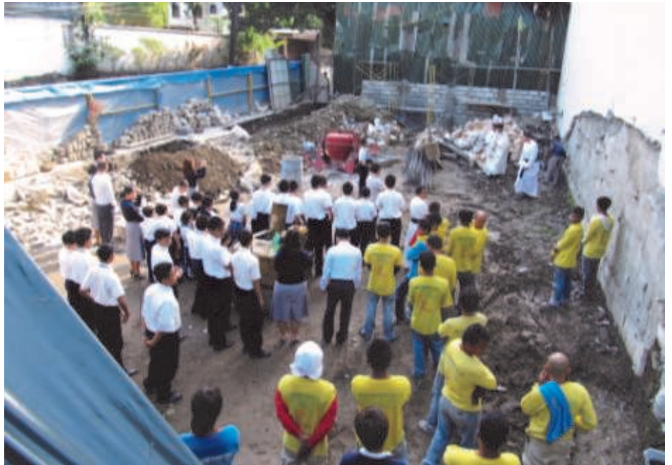
Blessing of the building site in the hope of many victories.
