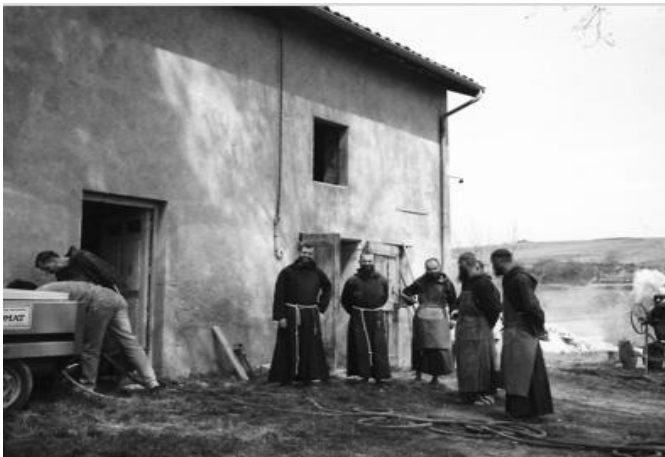
Building work on the vineyard house
